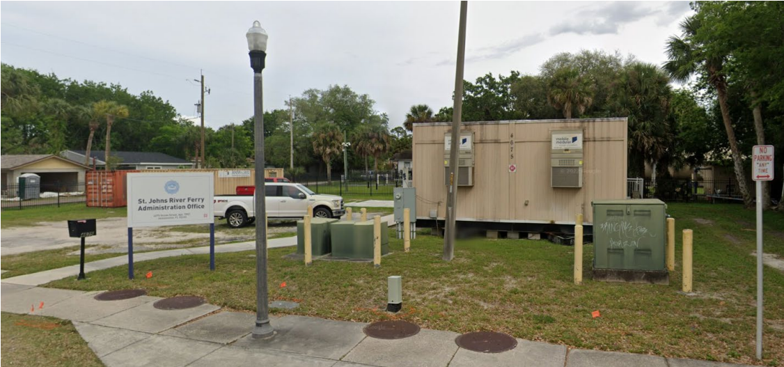
Figure 7-1 - Existing Ferry Administration Building
