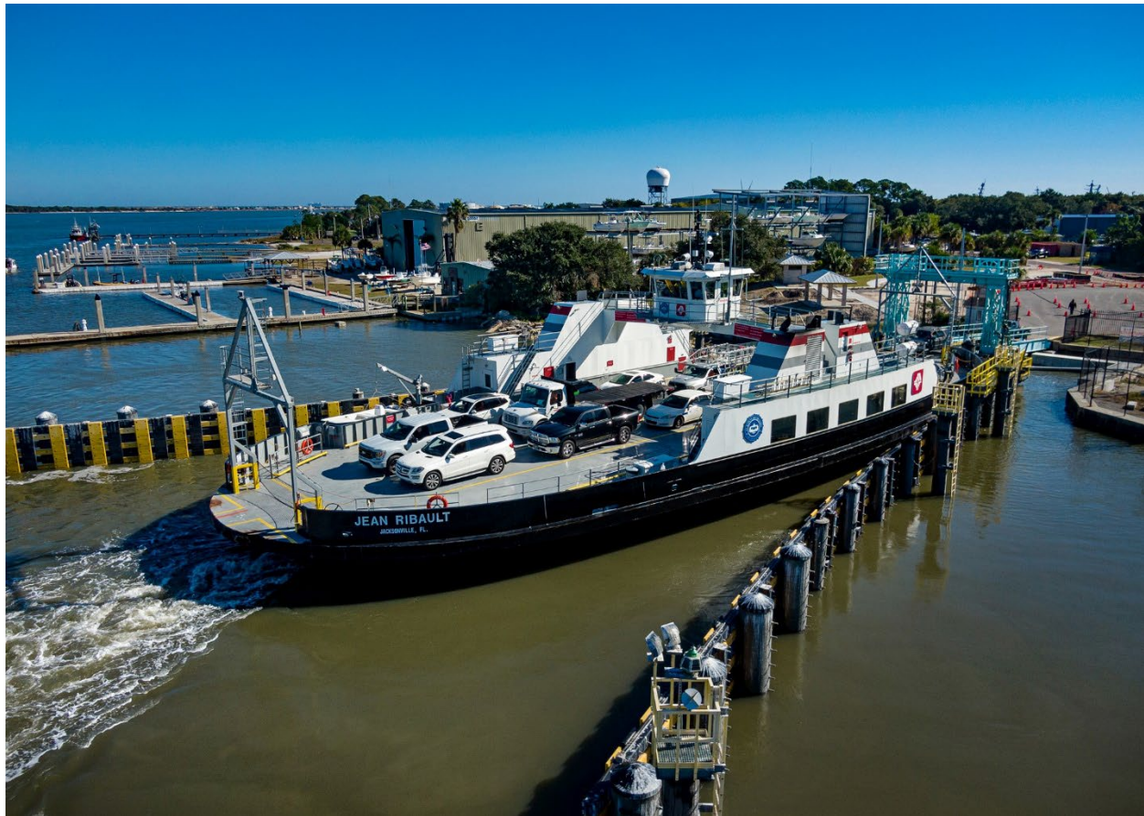
Figure 3-3 - View of Mayport Slipwalls after Phase IV
